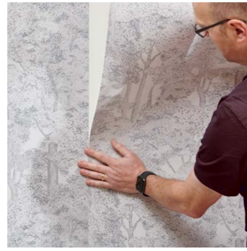
Step 3: Apply wallpaper onto the wall, smoothing out any lumps and bumps as you go. Make sure the pattern matches where each section meets
