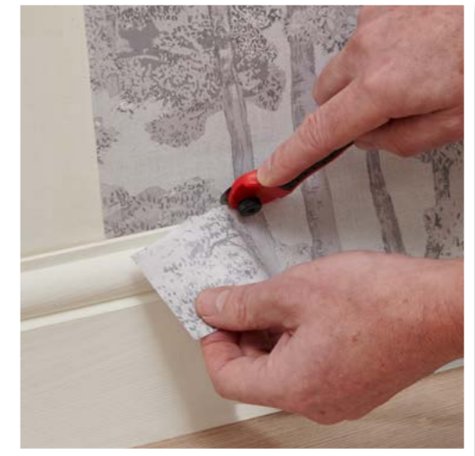
Step 4: Trim any excess wallpaper from the top and bottom
