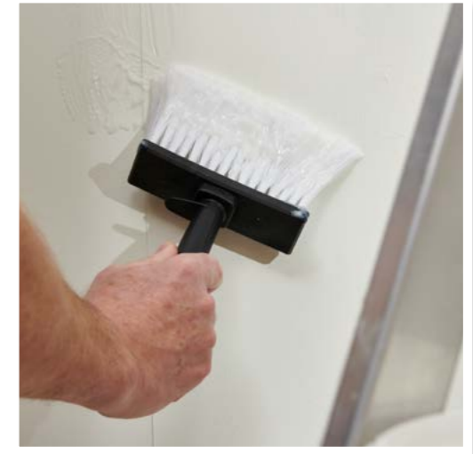
Step 2: Apply wallpaper paste to the section of wall you're about to cover
