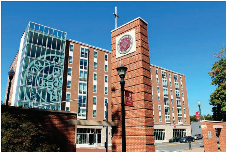
IONA COLLEGE RECENTLY OPENED ITS NEW NORTH AVENUE RESIDENCE HALL.
