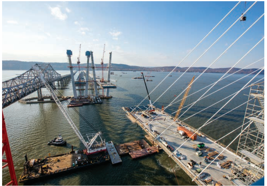
Left: With a lifting capacity of 1,900 tons, the I Lift NY crane is one of the largest floating cranes of its kind.
