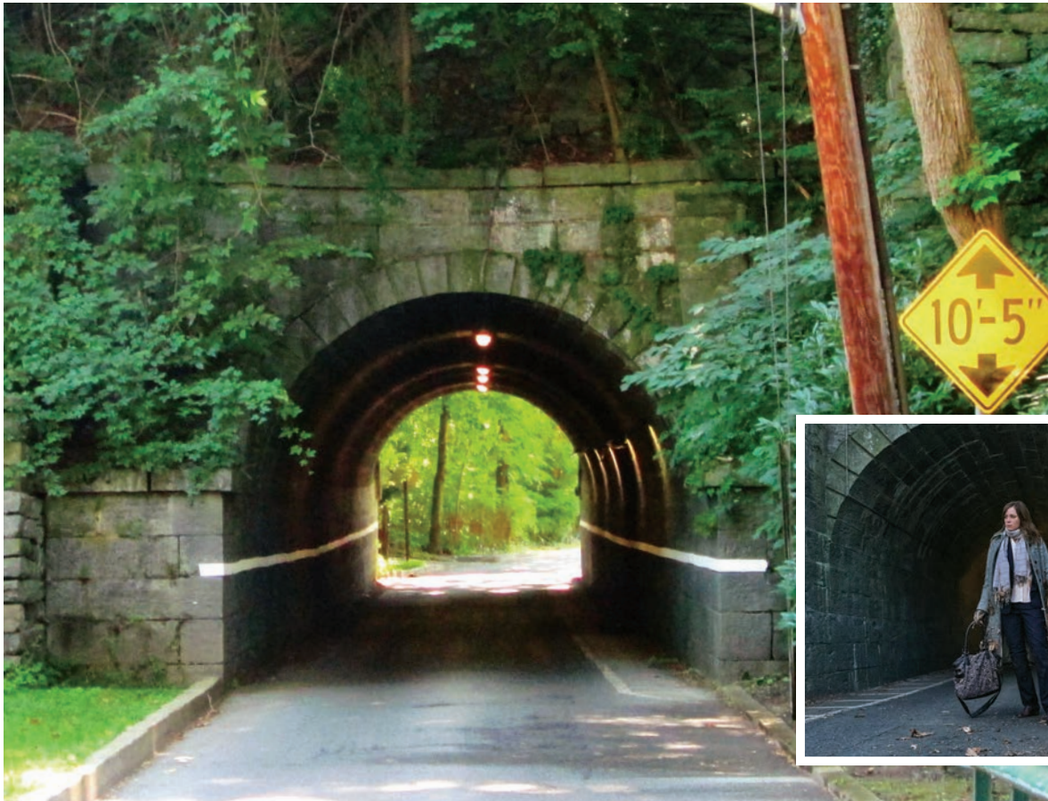
Left: Irvington's Station Road tunnel is the setting for a series of eerie scenes in the thriller The Girl on the Train ; below: Emily Blunt plays the film's troubled main character, Rachel Watson.
