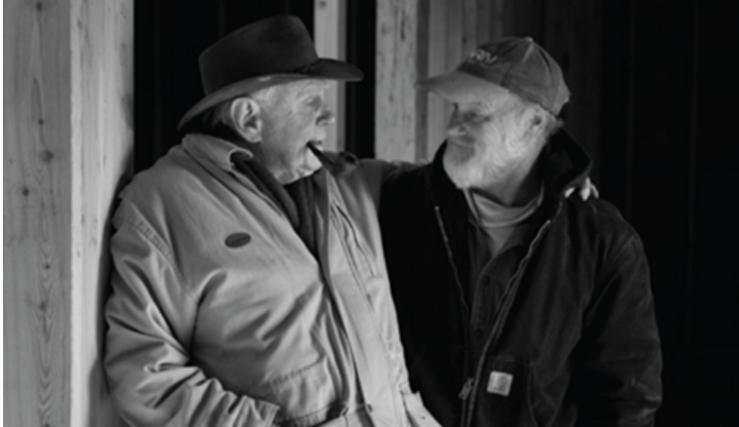
Raymond Plank with son Mike Plank at the construction site of the Raymond Plank Library and Center for Land Stewardship, 2012.
