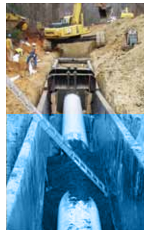
Trench box and backfilling.
