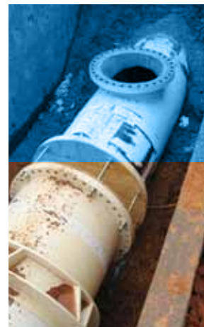
Manway for maintenance.
