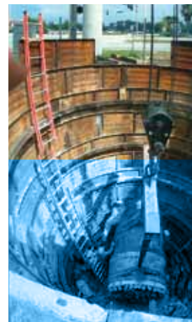
Receiving pit for 66-inch microtunnel.
