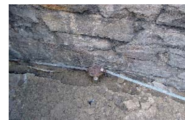
The tunnel was complete with electricity and light.
