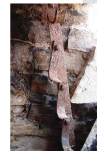
And looking west. The rusted hooks on the right-hand wall (and in the close-up to the left) held water pipes.
