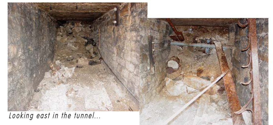
And looking west. The rusted hooks on the right-hand wall (and in the close-up to the left) held water pipes.
