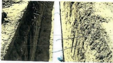
Environmental Infrastructure Loans
