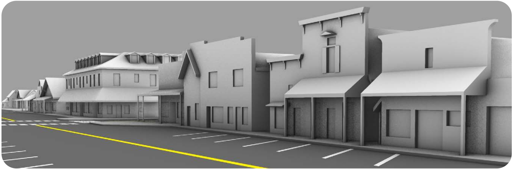
▲ Main Street looking East
