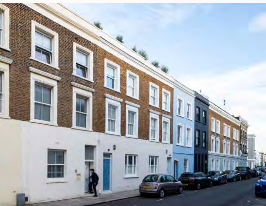
Princedale Road, certified as a Passive House // Photos by Adam Parker
