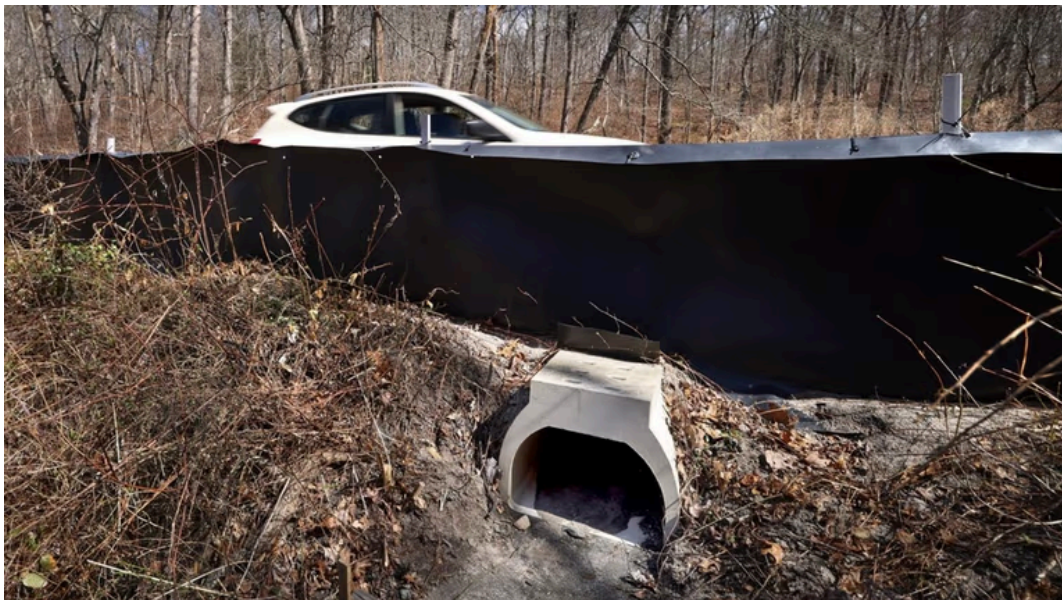
The Middle Island frog tunnel, installed so the amphibians could safely travel from one vernal pool to another. Credit: Newsday/John Paraskevas
