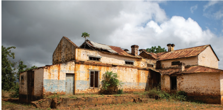
In Neno, Malawi, PIH built a new district hospital (right) in 2007 to replace the old building (left).
