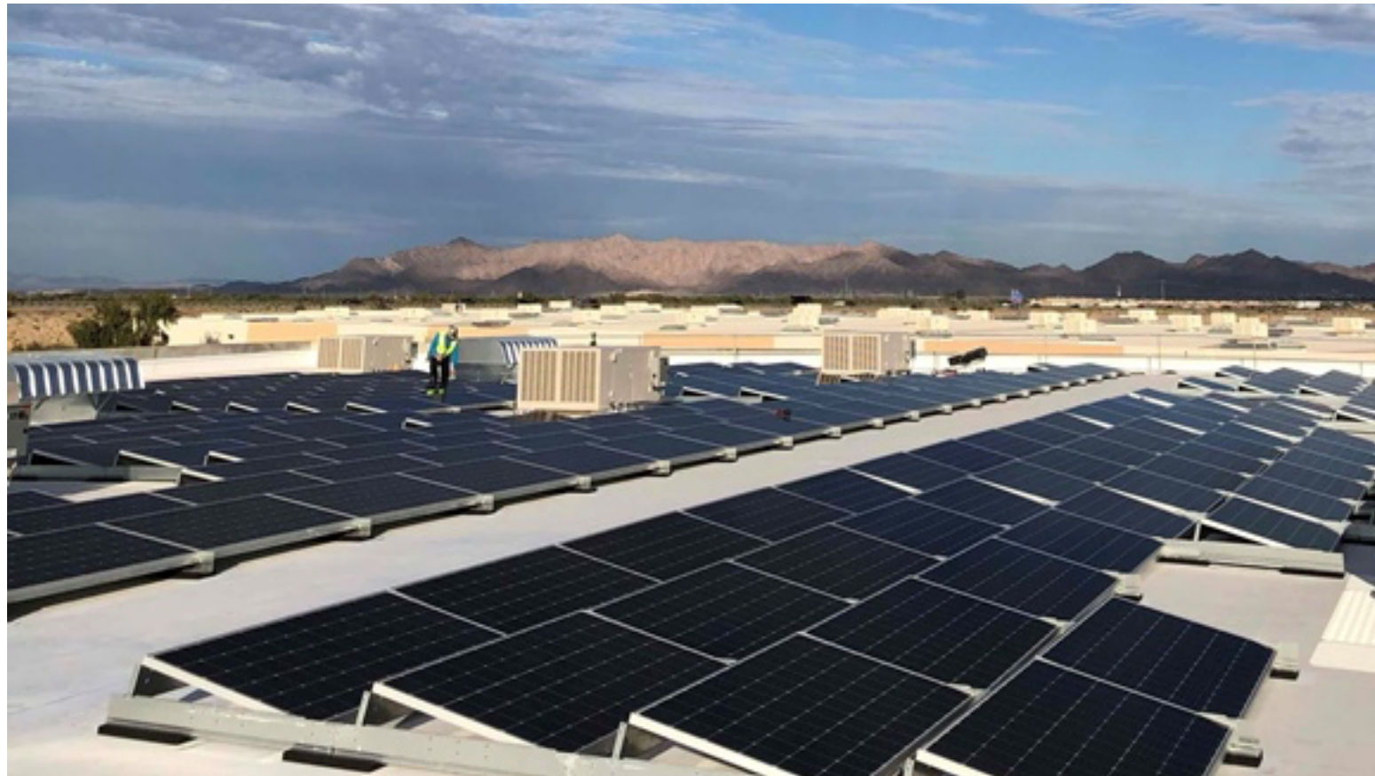
Rooftop solar installation at our new sales center in Yuma, AZ
