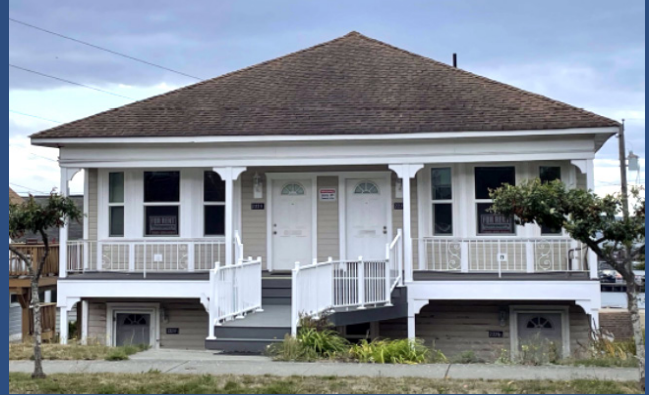
This fourplex in Everett, Washington, is an example of a house-scaled, four-unit building type that HB 1110 requires Washington cities to allow.
