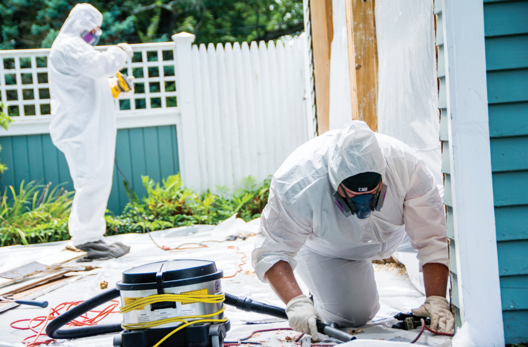
Photo by Mark Wilson | A crew with Alpine Environmental in Chelmsford, Mass., demonstrates proper lead containment on a home's exterior.
