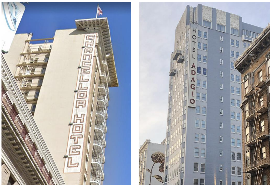
Chancellor Hotel and Hotel Adagio, two large-scale hotel projects in which Arthur and Oliver were involved.
