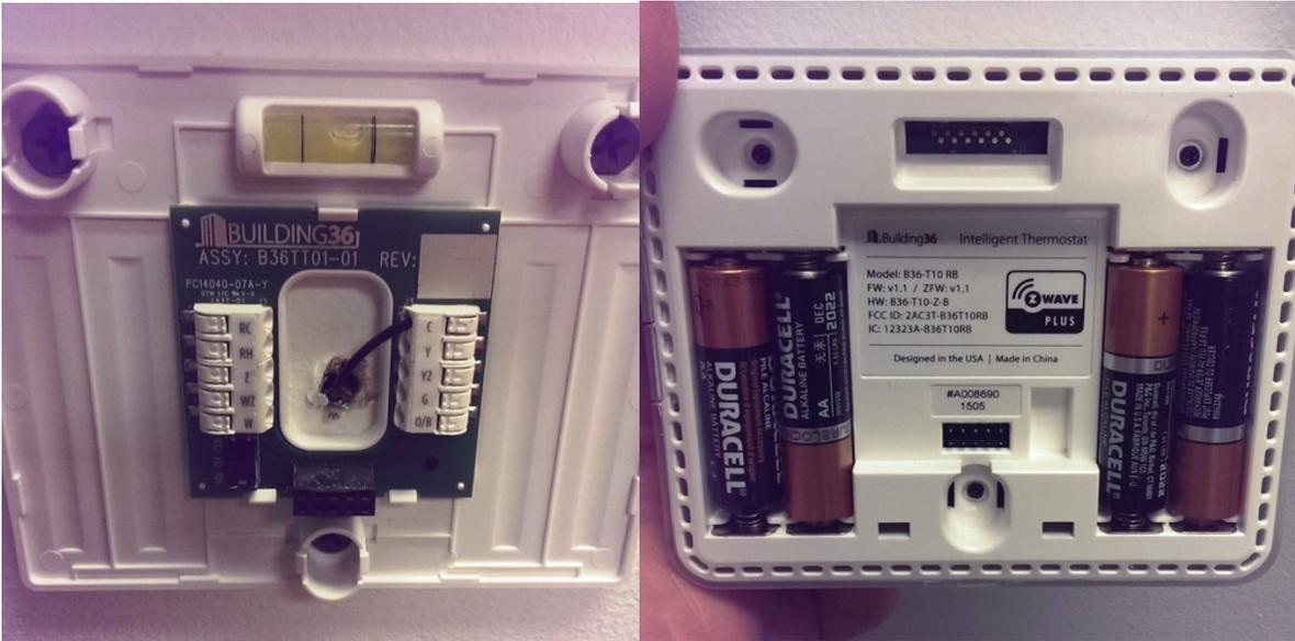
2. Remove the old batteries from the thermostat body.
