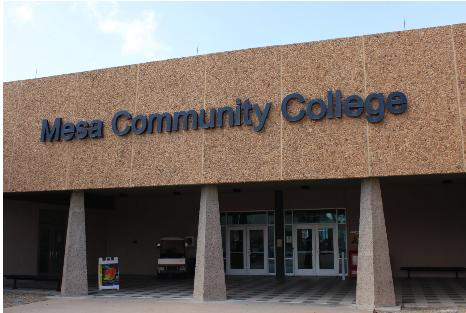
The front entrance to the MCC Library on the Southern and Dobson campus on Feb. 22, 2023. (Photo by Jordan Bell)
