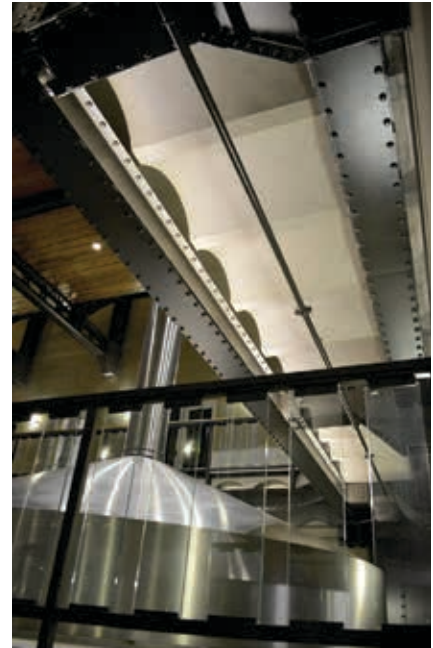
Scalloped precast ceiling in brewhouse.
