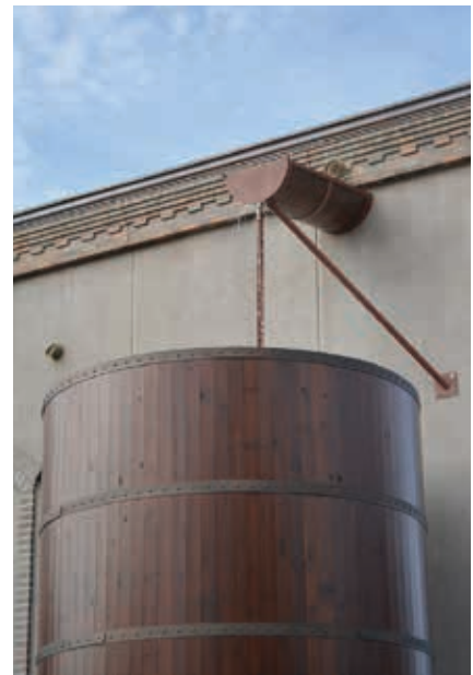
Architectural precast walls and rainwater collection outside warehouse.
