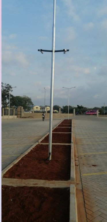
CCTVs on roads
