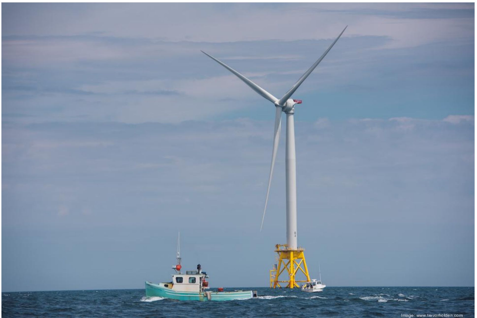
Block Island Wind Farm. Courtesy photo.
