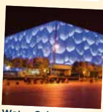
Water Cube National Aquatics Centre
