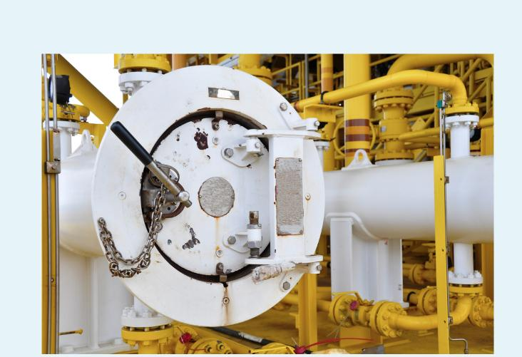
When pigging a gas pipeline, opening the pig launcher or the pig receiver portion of the line will often emit a portion of trapped gas.
