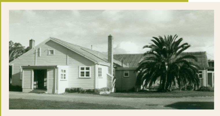
Top: The Bernard Chambers Building at Massey was the veterinary clinic during the 1960s. Above: This building served as the temporary veterinary laboratory
