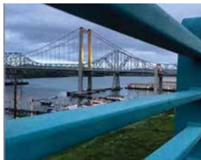
The Alfred Zampa Memorial Bridge @stikki_nikki
