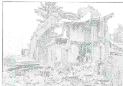
THE CLOISTERS APARTMENTS COMING DOWN LAST SPRING
