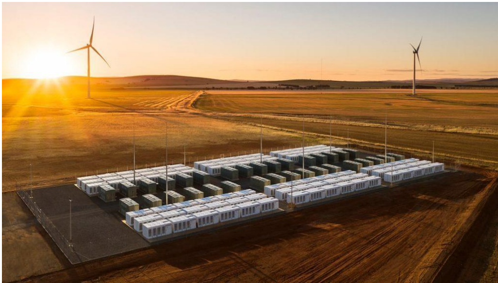
Tesla's Hornsdale Power Reserve is the world's largest lithium-ion battery (Source: Hornsdale Power Reserve)
