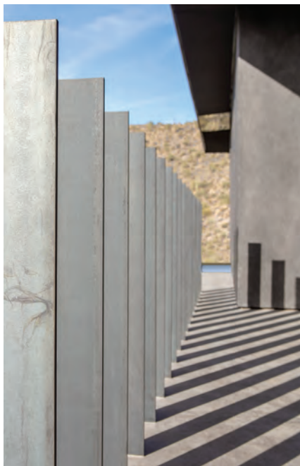
Shadows play off a steel plate guard rail along the southern edge of the house, creating a sundial effect.
