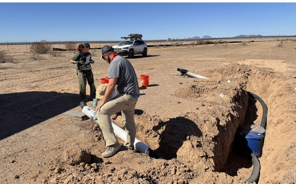
Wild at Heart and Longroad Energy volunteers build an artificial burrow at the Sun Streams solar complex.
