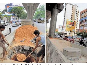
Workers dig to build a tank for rainwater harvesting between Metro pillars. (R) The completed tank. DH FILE PHOTO
