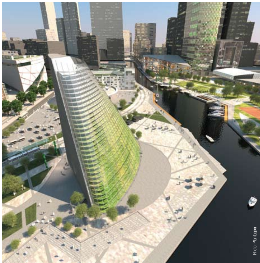
Plantagon's innovative cone-shaped design will allow optimum light to reach the produce growing inside, resulting in 10 harvests per year
