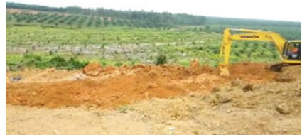
The company taking the Laterite soil. (Photo by WALHI Central Kalimantan)
