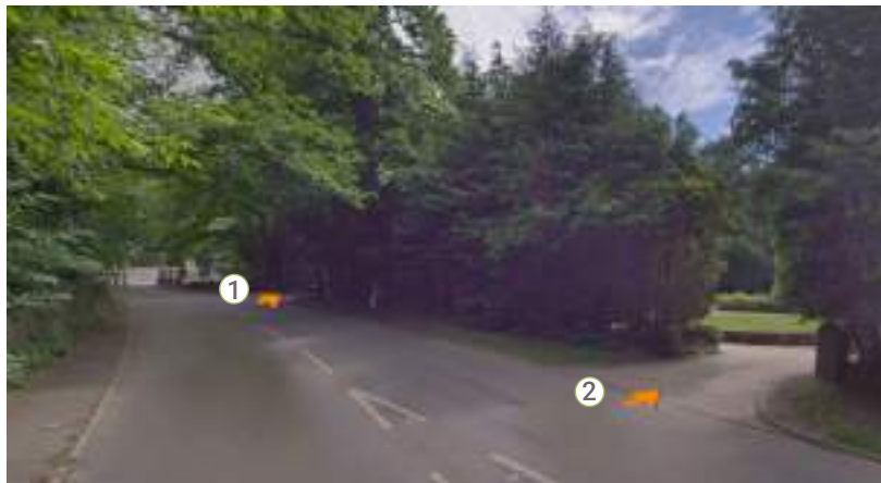
› Views of existing Site access from Deepcut Bridge Road
