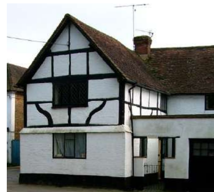
③ The Old House, Portsmouth Road - Listed building, Grade II
