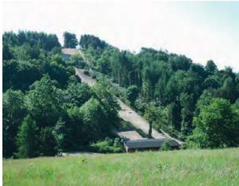
Pontypool dry ski slope is a notable leisure facility
