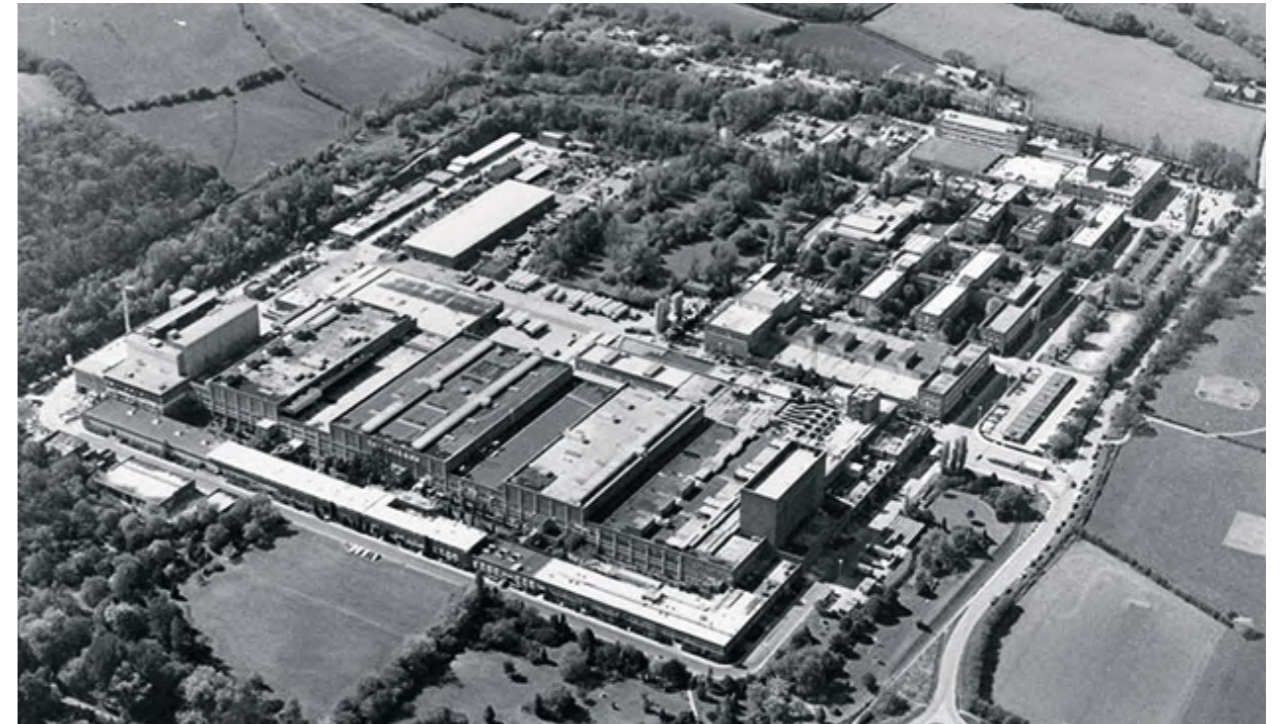
Aerial photograph of site and former Nylon Spinners Factory in the foreground
