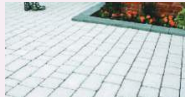
Example of permeable paving solutions for access drives
