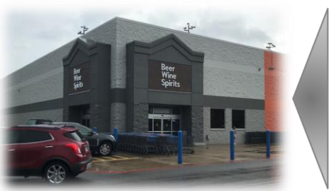
Outside entrance view
