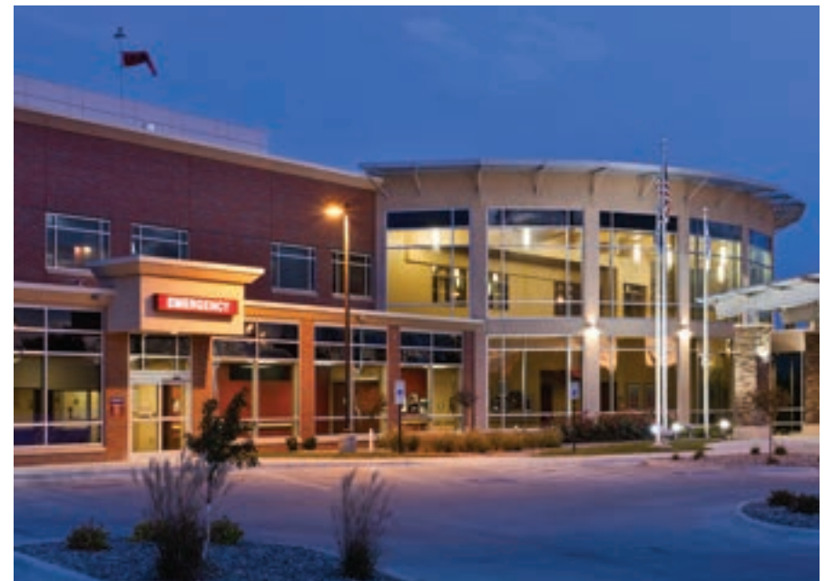
Memorial Community Hospital Addition/Renovation, Blair, NE
