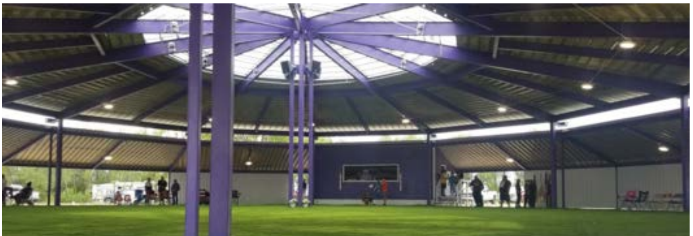
Lucky Mound Celebration Grounds Roof Structure for the Three Affiliated Tribes: Mandan, Hidatsa, and Arikara in Parshall, ND
