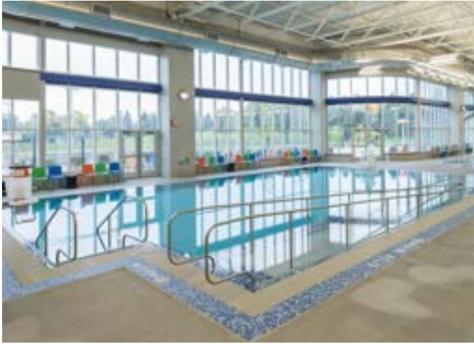
Warm-water therapy pool with dual step and ramp entry at Midco Aquatic Center, Sioux Falls, SD
