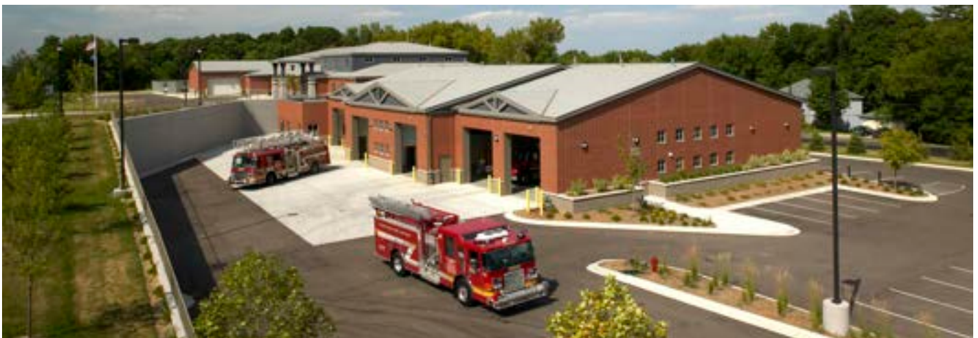
Excelsior Fire District/South Lake Minnetonka Police Department Joint Public Safety Center in Shorewood, MN
