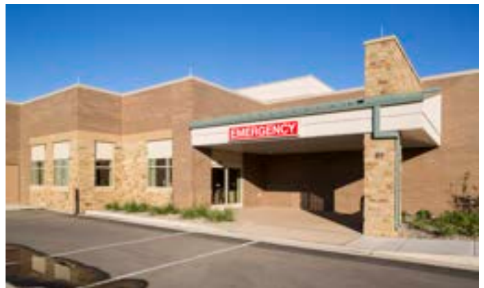
A TSP-designed, USDA-funded project: Madison Regional Health System Replacement Hospital & Clinic, Madison, SD
