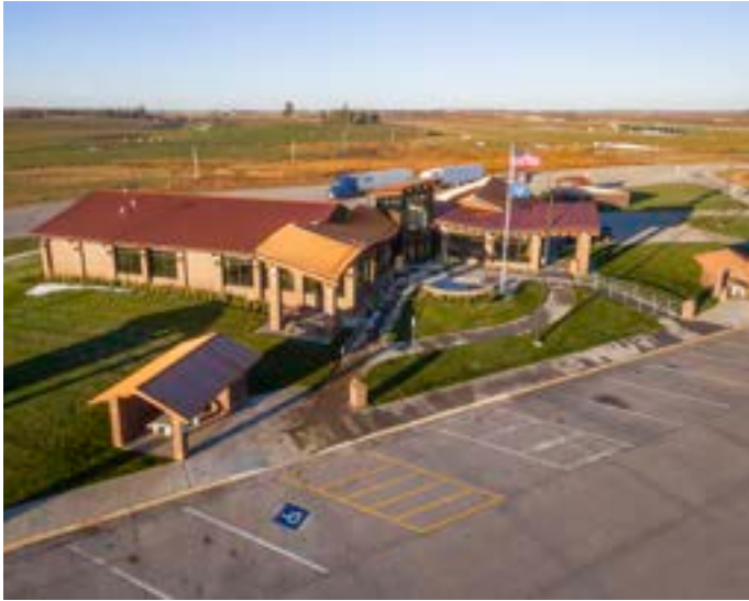
South Dakota Department of Transportation Welcome Center, a TSP + Confluence project at the Interstate 29 Wilmot exit
