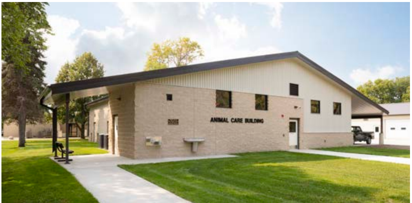
This page: Bramble Park Zoo Animal Care Building, a TSP project for City of Watertown
