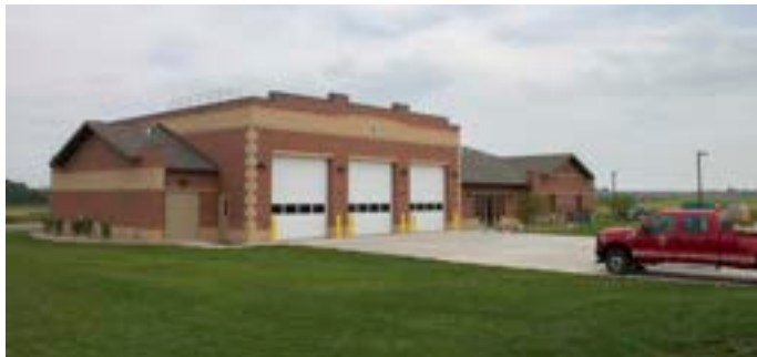
Streetfront (top) and rear views of City of Sioux Falls Fire Rescue Station 11, Sioux Falls, SD
