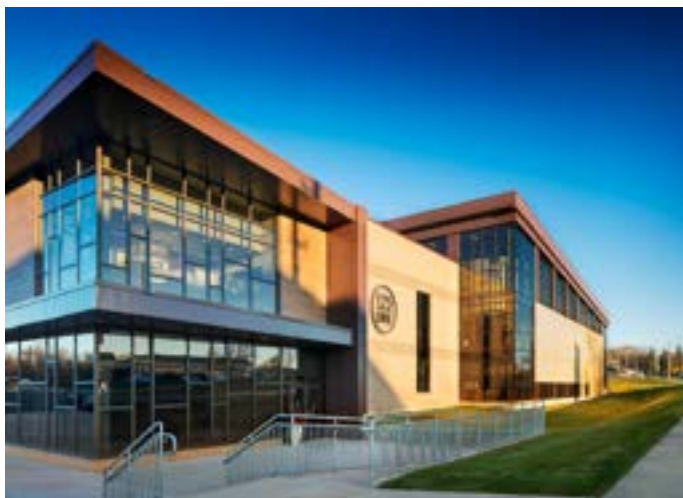
Recreation Center Addition/Renovation & New 125 LIVE Center for Active Adults, a TSP + MBJ project for City of Rochester, MN
