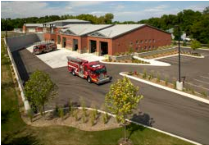
Excelsior Fire District/South Lake Minnetonka Police Department Joint Public Safety Center in Shorewood, MN, a TSP-designed project teamed with David Rey of Bolton & Menk
