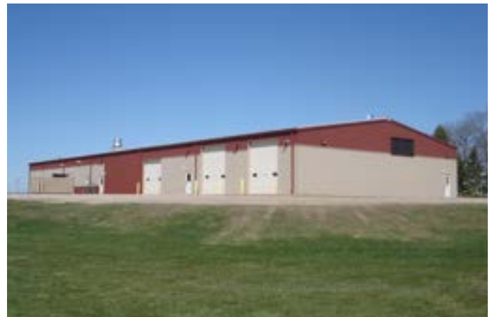
City of Hartford Fire & Rescue Station, a pre-engineered metal building (PEMB) completed Spring 2012 in Hartford, SD, at a cost of $88 per square foot (roughly $110/sf in 2020 dollars)
