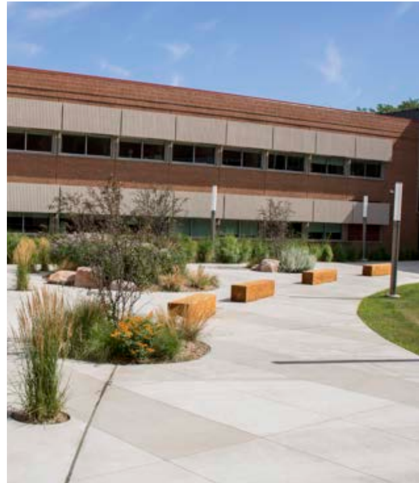
Augustana University Froiland Science Complex, a TSP + Confluence + Sayre Associates project in Sioux Falls, SD
