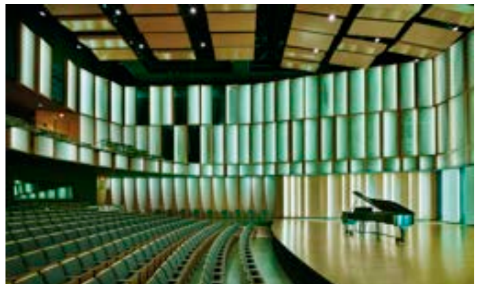
One venue, many moods: The Kracum Performance Hall within Carleton College Weitz Center for Creativity, Northfield, MN. Wood panels and metal mesh compose the acoustically transparent visual surround, concealing color-changing LED strips.
