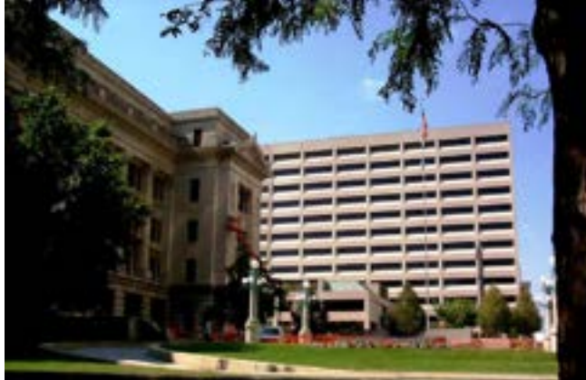
Existing Hall of Justice courthouse and offices tower
