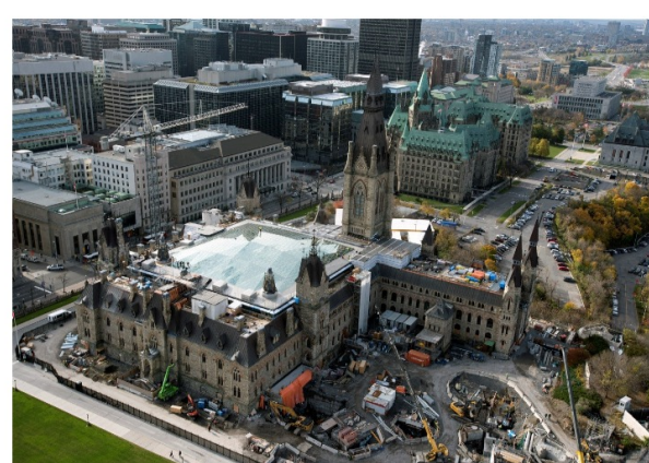
West Block Under Construction
