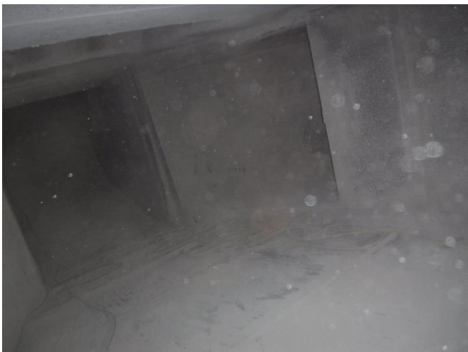
INT 9 – View of duct
