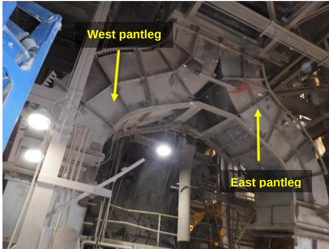
EXT 29 – Duct pant leg
