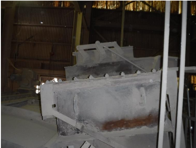
EXT 17 – Heavy oxidation
