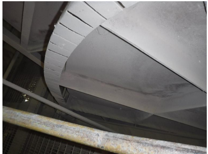
EXT 14 – Underside of the duct
