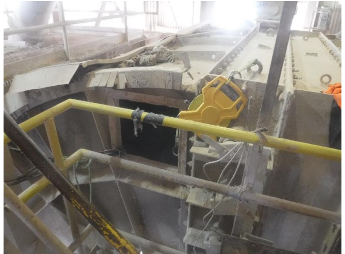
INT 2 – Opening to duct
