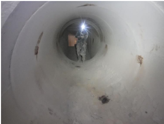
INT 37 – Looking through duct
