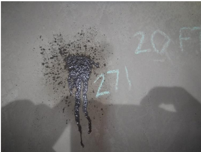
INT 25 – 20'± – View of duct wall
