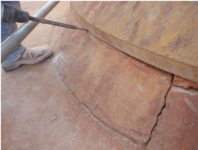
IMG 3 – Curb being chiseled out
