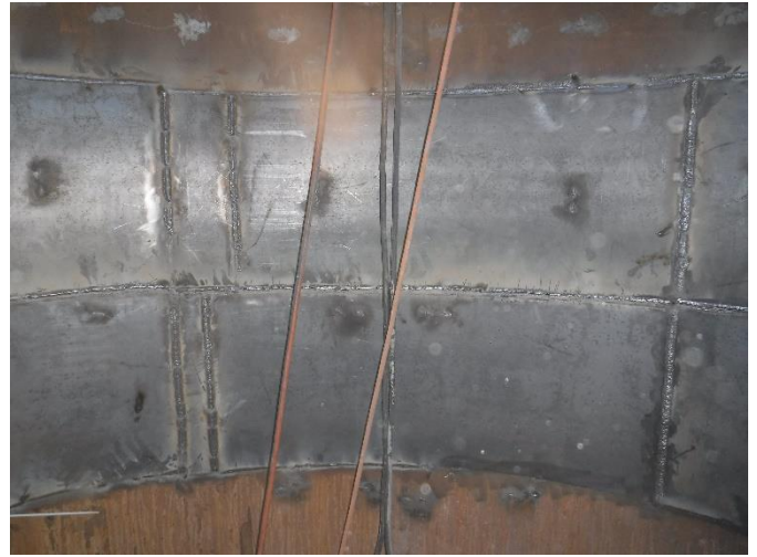
IMG 22 – View of interior after plate installation
