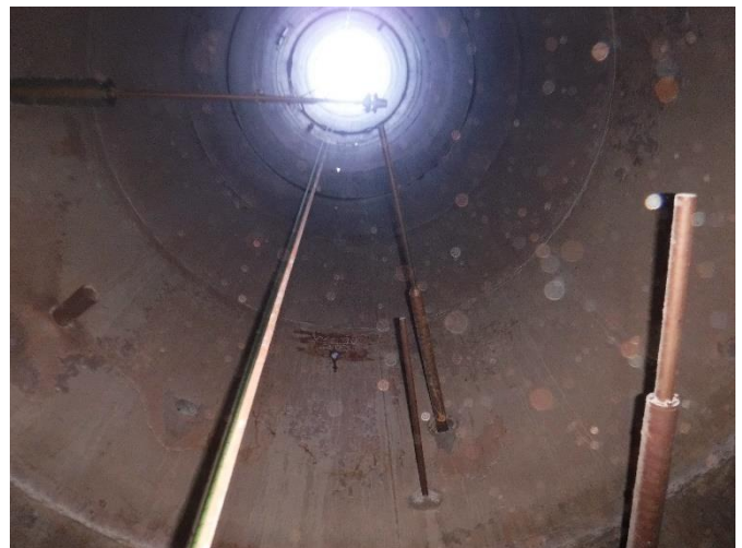
INT 40 – W EL. 85± – Test ports & probes
