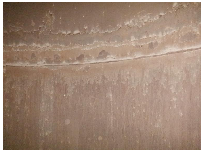
INT 22 – E EL. 150'± – Buildup on flanged joint
