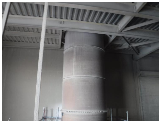
EXT 32 – 7 th Floor – Floor penetration point
