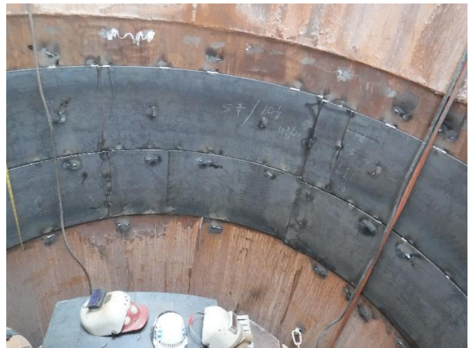
IMG 20 – View of interior after plate installation
