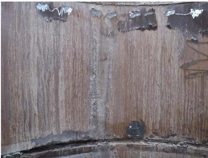
IMG 19 – View of interior before plate installation
