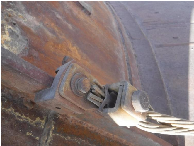
EXT 13 – Roof – LPS conductor
