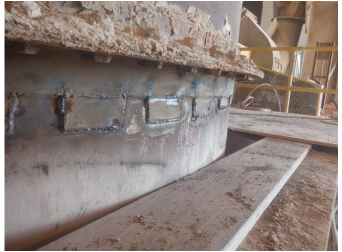
IMG 30 – View of stack after holes repaired
