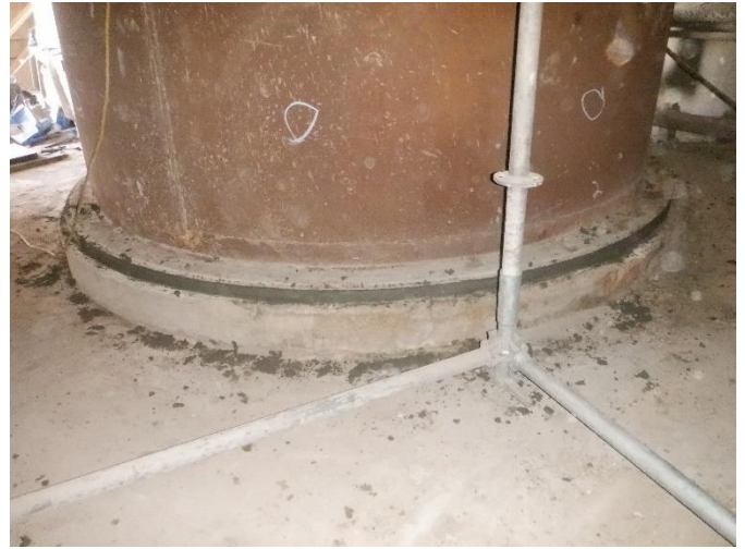
IMG 14 – Reconstructed base after repair process
