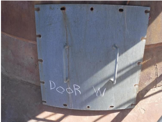
EXT 5 – Roof – Access door removed from access opening for inspection purposes
