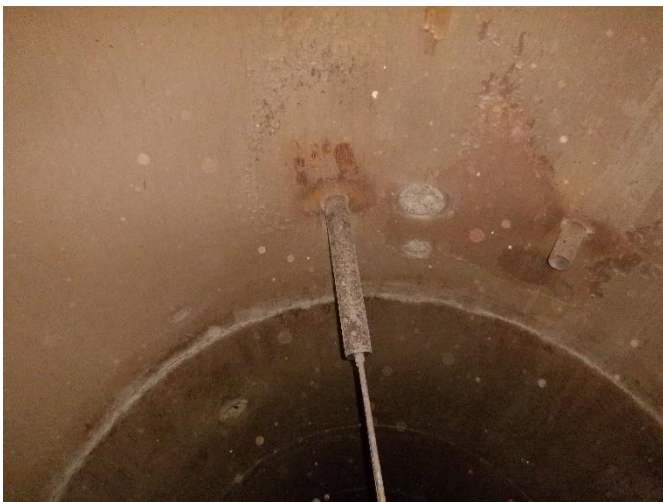
INT 39 – E EL. 85± – Port openings and test probe
