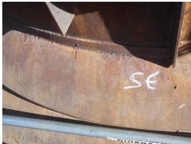
EXT 18 – Southeast of rain hood
