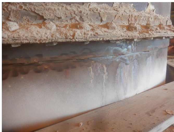
IMG 26 – Buildup removed
