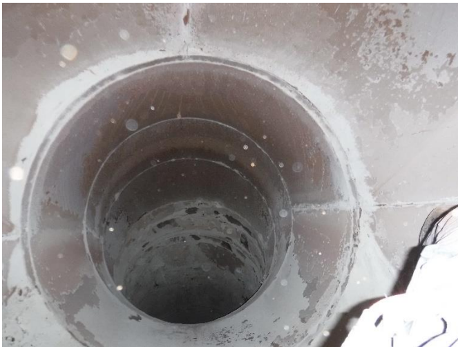
INT 49 – EL. 20'± – Interior of breeching duct
