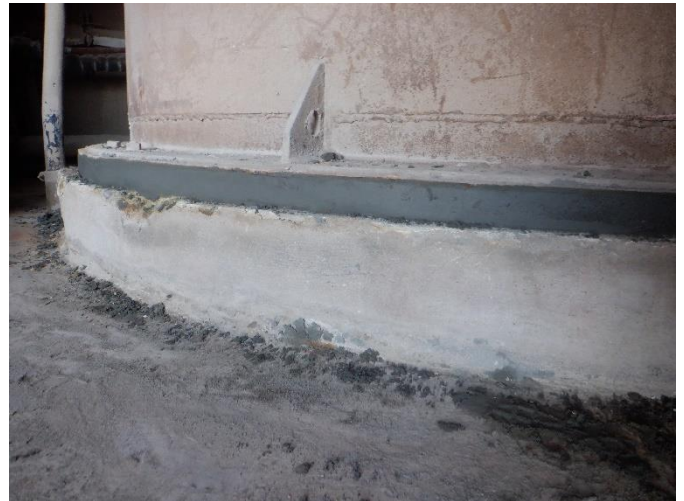
IMG 12 – Reconstructed base after repair process
