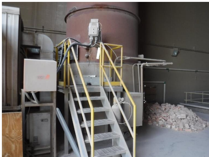
EXT 29 – View of test platform
