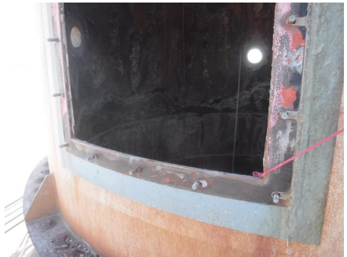
EXT 4 – EL. 200± – View of access door opening
