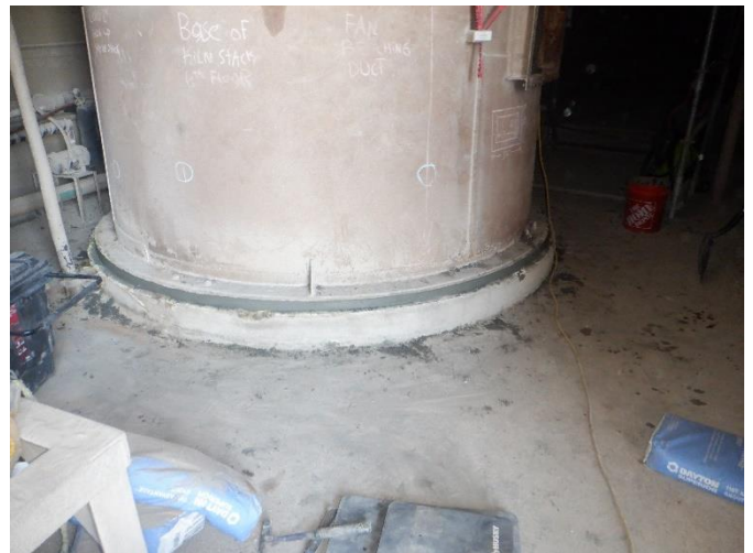
IMG 16 – Reconstructed base after repair process
