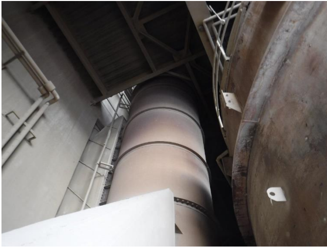
EXT 35 – 6 th Floor – View of penetration point
