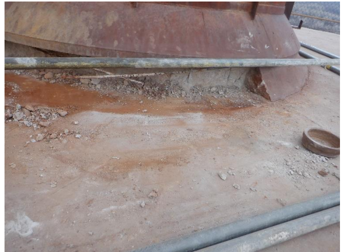
IMG 4 – Curb after damaged section removed
