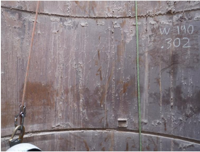
IMG 21 – View of interior before plate installation
