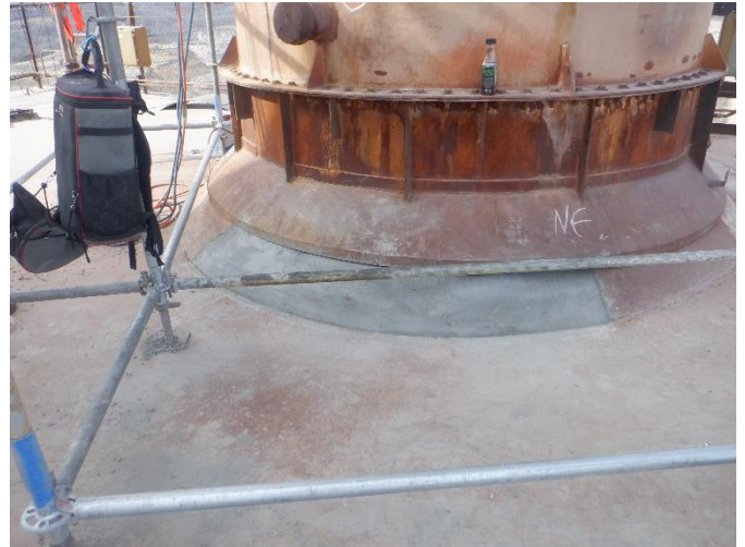
IMG 6 – Mortar after drying
