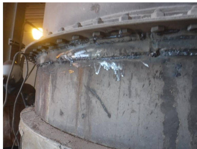
IMG 36 – Crack and weld sealed shut
