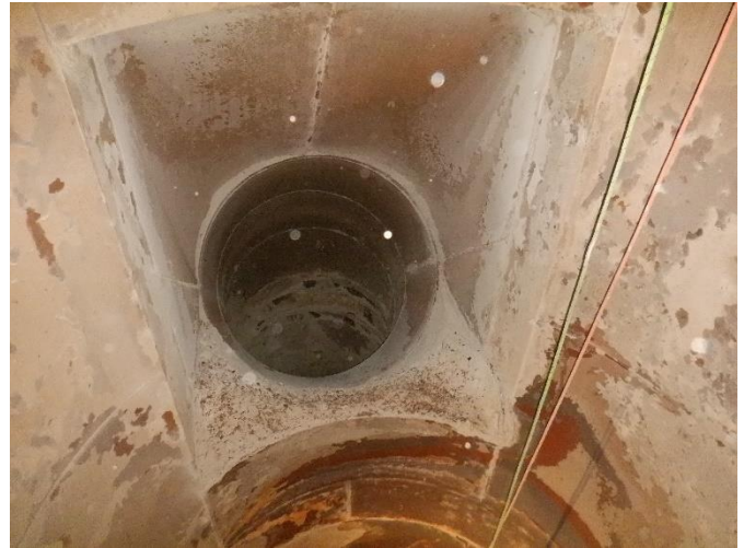
INT 48 – E EL. 20± – Interior of breeching duct
