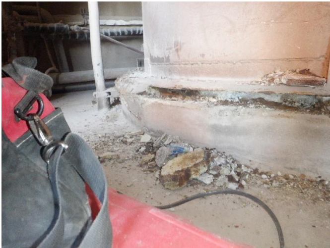
IMG 11 – Damaged sections of mortar removed
