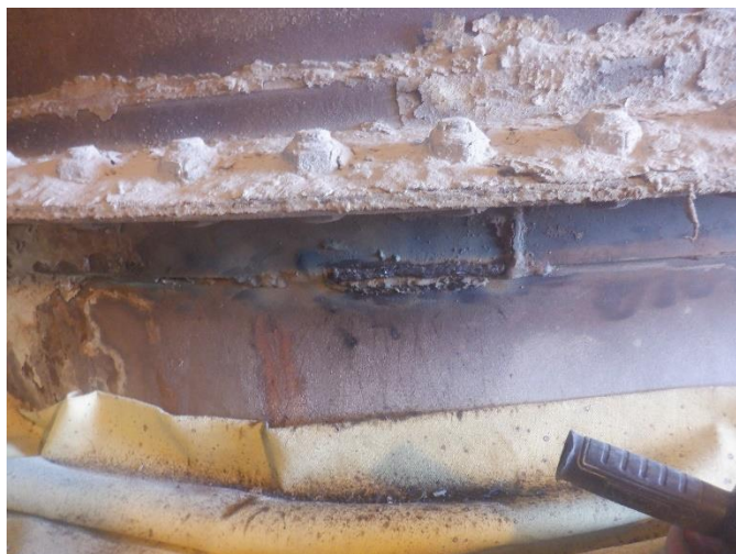
IMG 27 – Hole being welded shut
