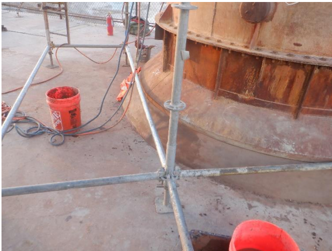
IMG 7 – Final view of curb repair
