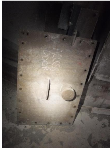
EXT 38 – Access door removed for inspection purposes
