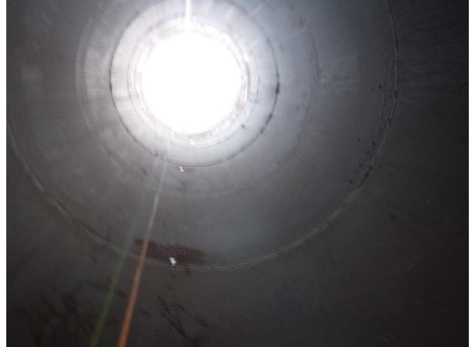
INT 18 – W EL. 160'± – Upward view of stack interior
