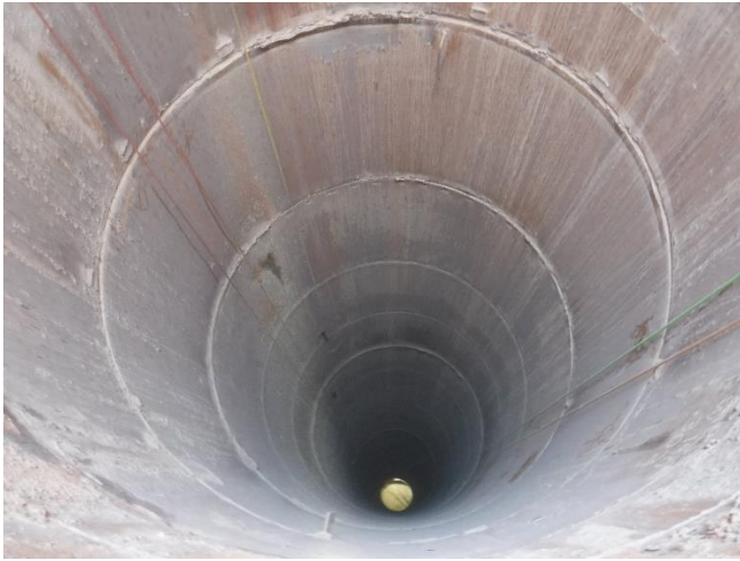
IMG 17 – View of interior before plate installation
