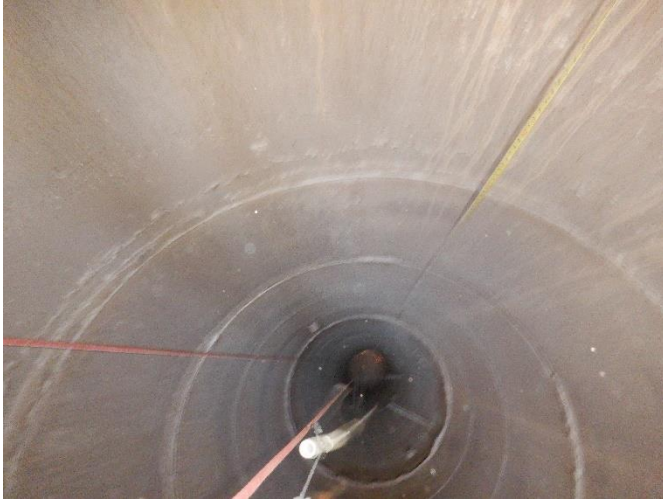
INT 17 – E EL. 160'± – Downward view of stack interior
