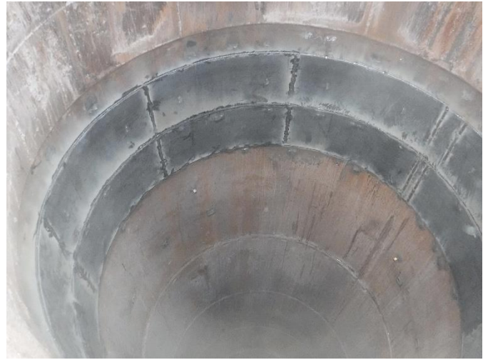
IMG 18 – View of interior after plate installation
