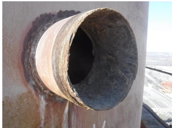
EXT 8 – Drop #1 EL. 70'± – Closeup on port
