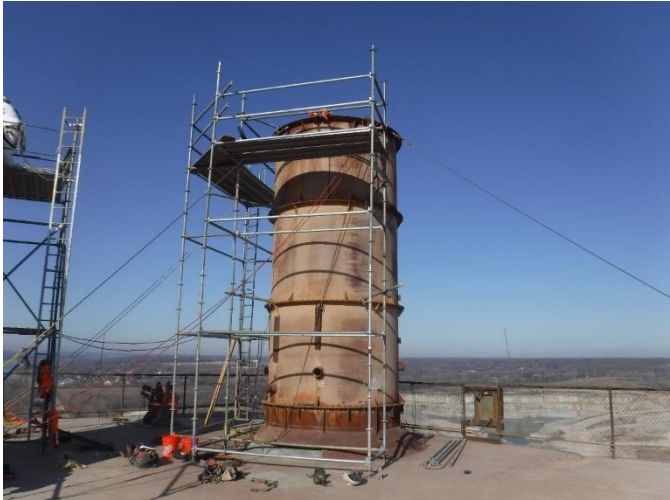
EXT 1 – View of the stack above the roof.
