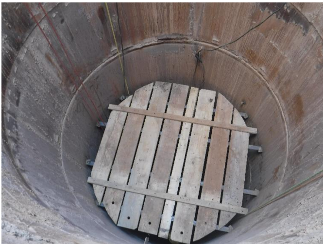
IMG 23 – View of interior before plate installation
