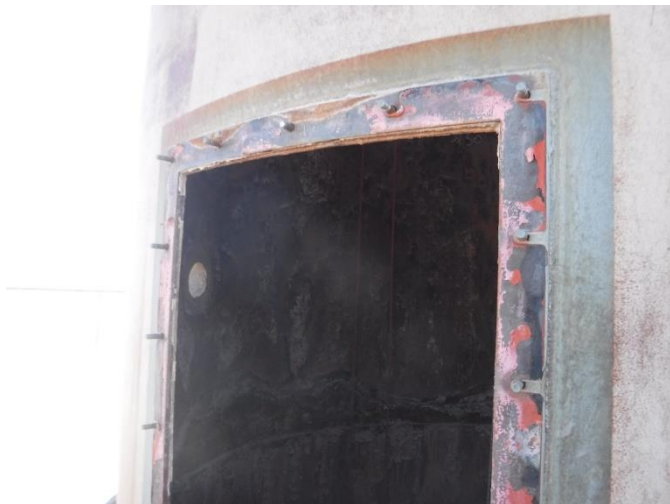
EXT 3 – EL. 200± - View of access door opening
