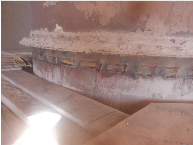
IMG 31 – View of stack after holes repaired
