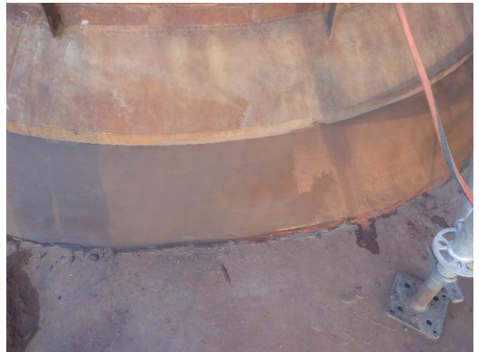
IMG 8 – Final view of curb repair
