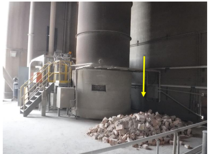
EXT 28 – 8 th Floor – Debris on Floor
