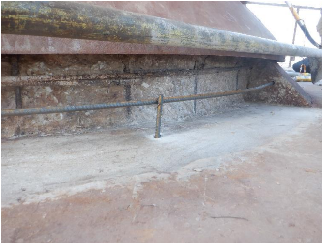
IMG 5 – New rebar installed
