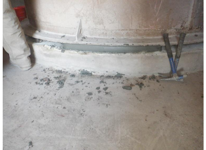
IMG 10 – Reconstructed base after repair process
