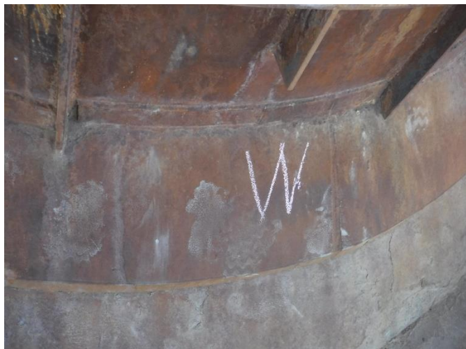
EXT 17 – Roof – West of rain hood
