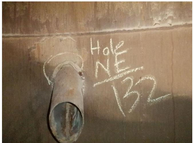
INT 26 – E EL. 140'± – Hole present in instrument port nozzle
