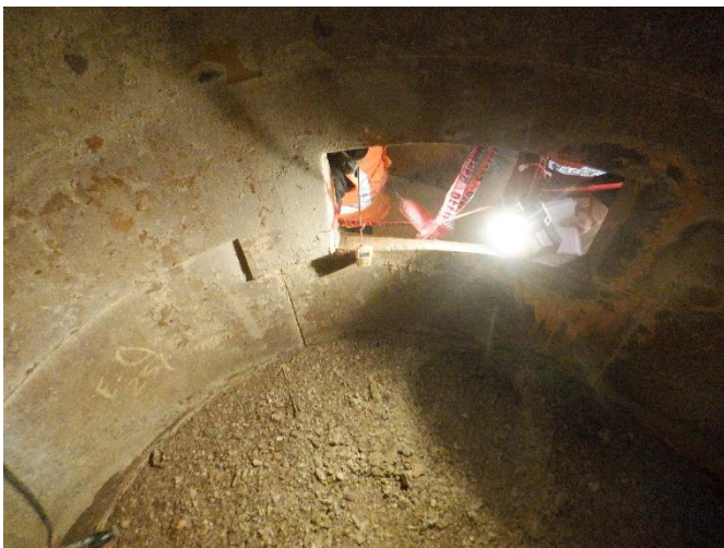
INT 51 – E EL. 0 ± – Stack floor and access opening
