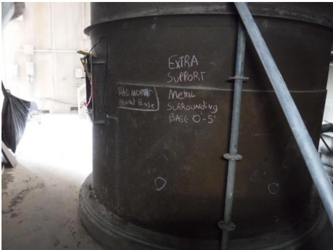
EXT 39 – View of stack
