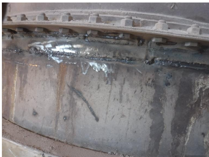
IMG 37 – Crack and weld sealed shut
