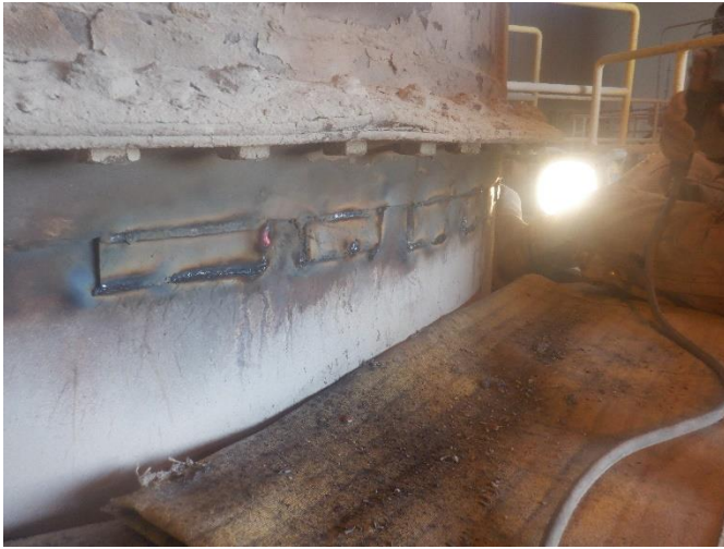
IMG 29 – View of stack after holes repaired
