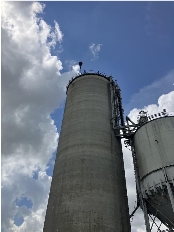
EXT 1 – Upward view of silo from the North side
