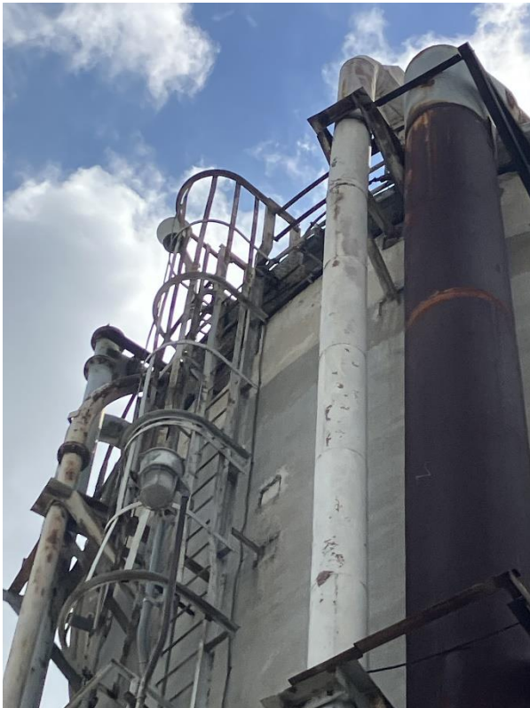
EXT 7 – View of silo from the west
