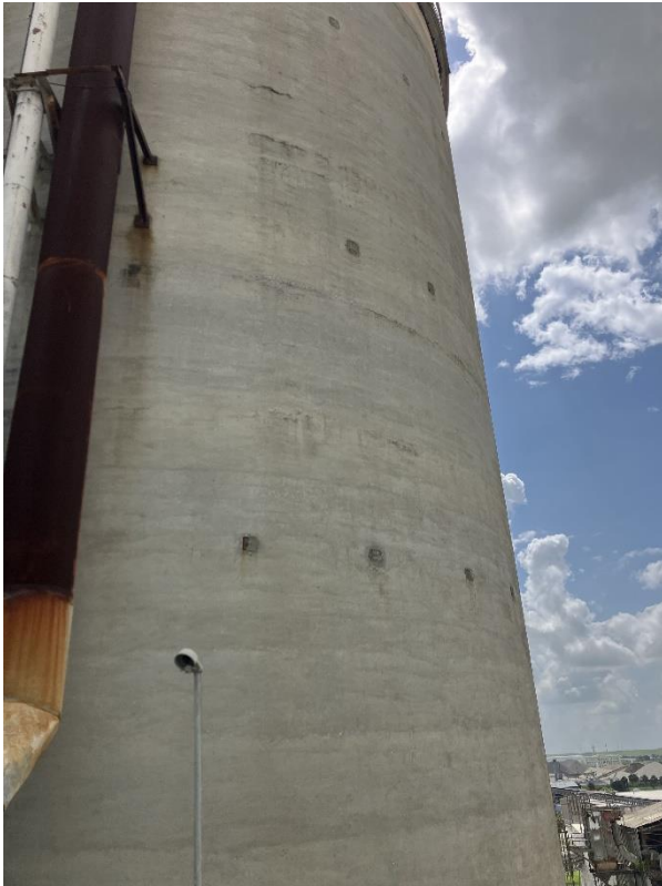
EXT 5 – View of silo from west side
