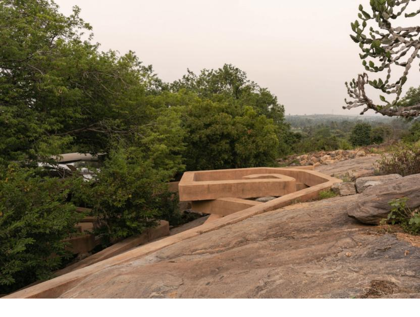
first attempt at building directly on to a rock face. We used a camouflage construction technique to blend the home into the landscape and keep it from hindering the natural beauty of its surroundings.' He gestures to the swirling walls, which are, in fact, precast beams, fashioned from debris, earth and discarded plastic bottles, which spiral up to parlay into a perfectly flat, polygonal glass roof.
